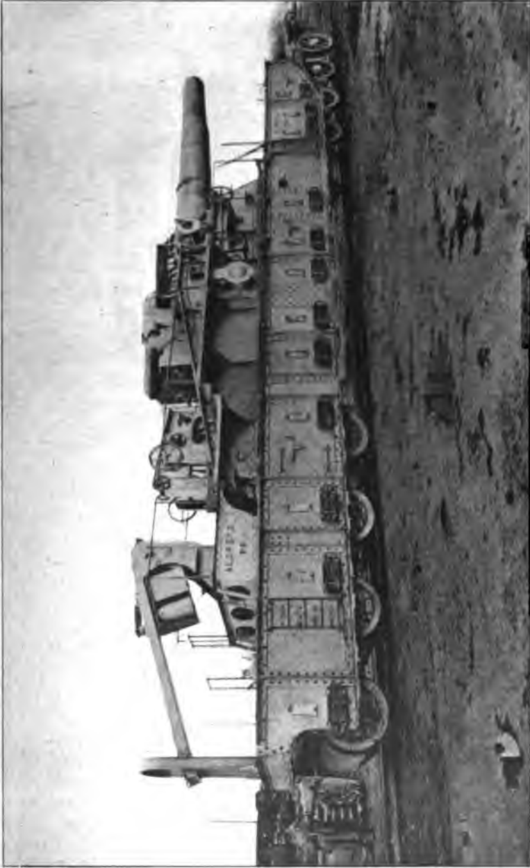
370-MM. FRENCH HOWITZER ON BATIGNOLLES MOUNT.
